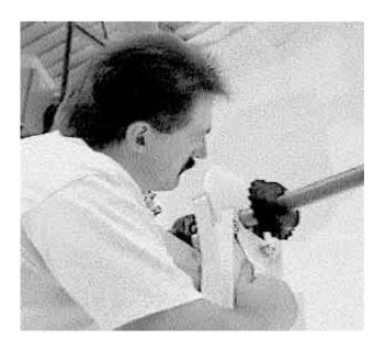
Hook the right channel onto the shaft just inside of the square channel-bearing. This channel with the control panel attached is quite heavy definitely a two person job. One person on the ground must hold the channel in place while the ladder person bolts it onto the bearing. Only install the bottom two bolts in each bearing at this time.
