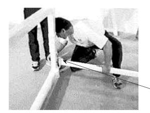
The *horizontal braces* are long rectangular tubing with L-shaped fittings welded to each end.
