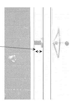
The *cable-guards* are short channel-shaped pieces with two long hooks that hold them onto the cables.
