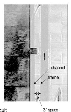
Handy-Tip: If this alignment is off, it may be difficult to lock the chrome ring on the adjuster pipe to the channel - the spacing will be wrong.
