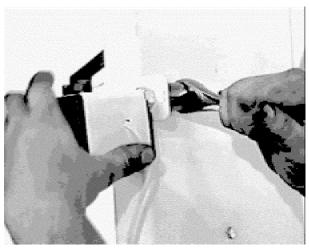
The *counter* is in a small box with a stud and protruding wires.
